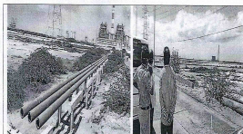
Partially completed ash slurry pipelines for the M/s.NCTPS Stage-III
