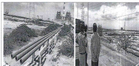
Partially completed ash slurry pipelines for the M/s.NCTPS Stage-III
